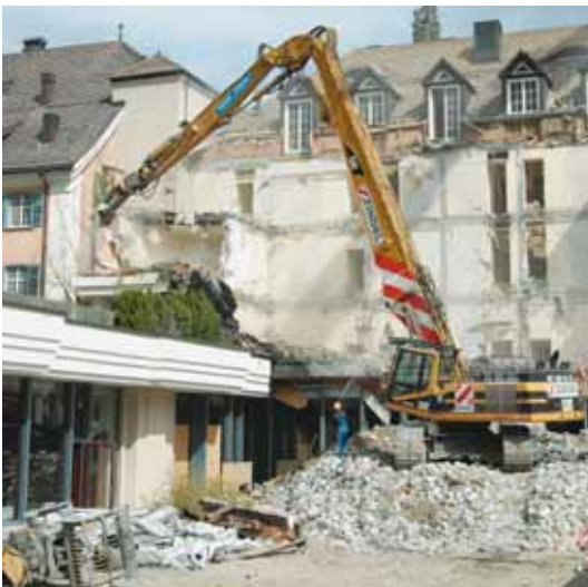
A long-arm excavator removes the rest of the Middle House.
